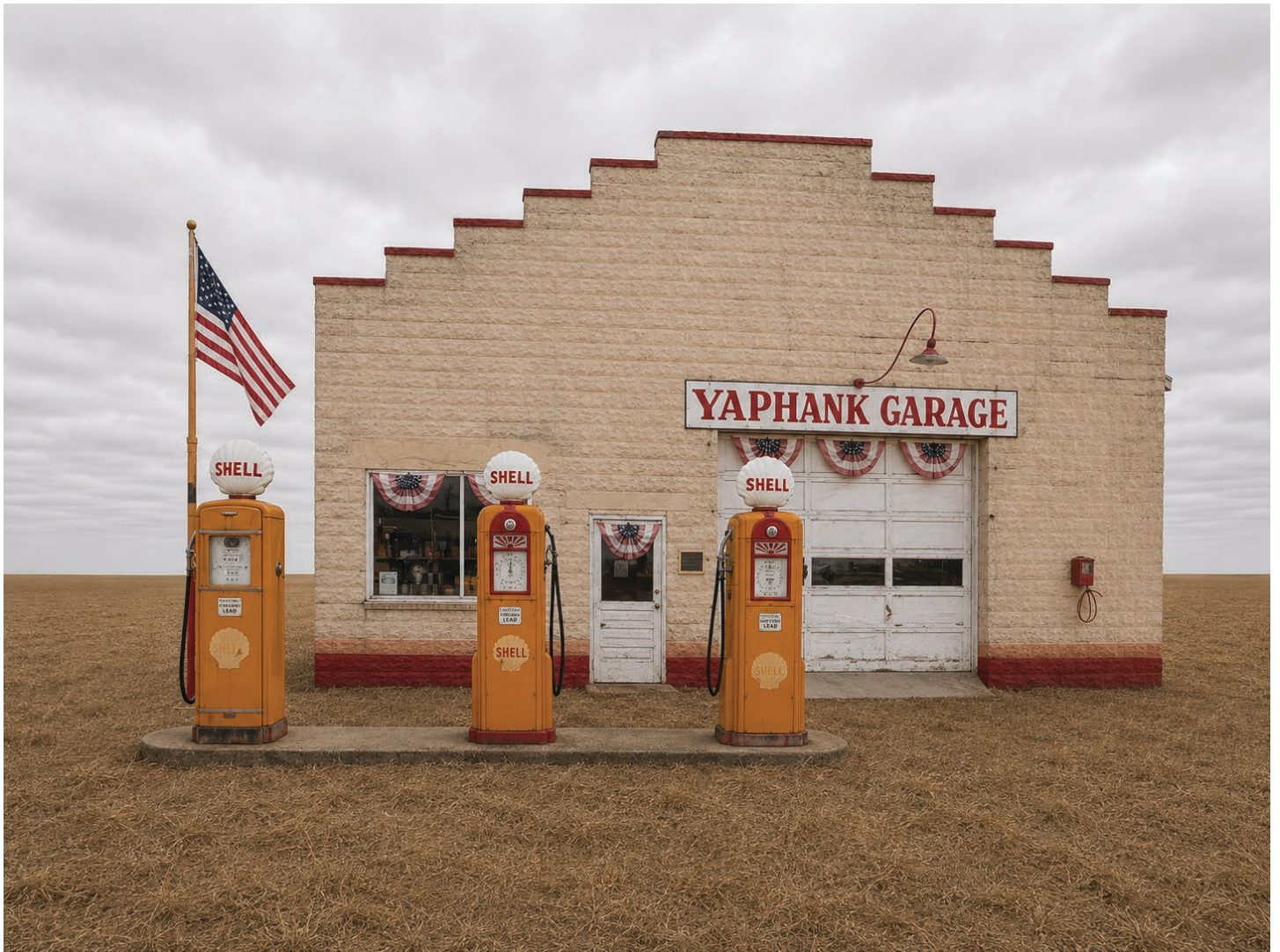
Yaphank Garage — Shell Pumps
