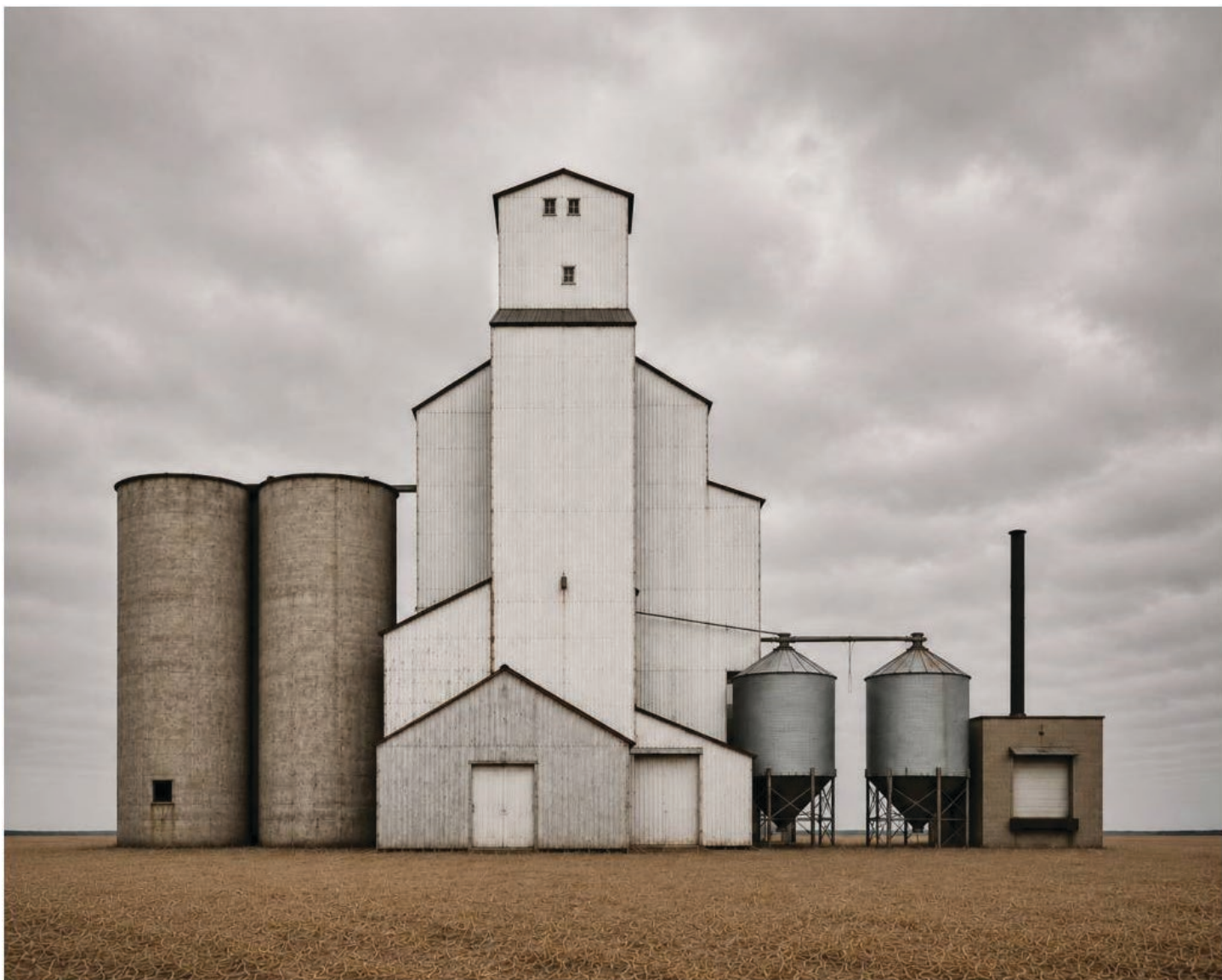
Grain & Feed Silos
